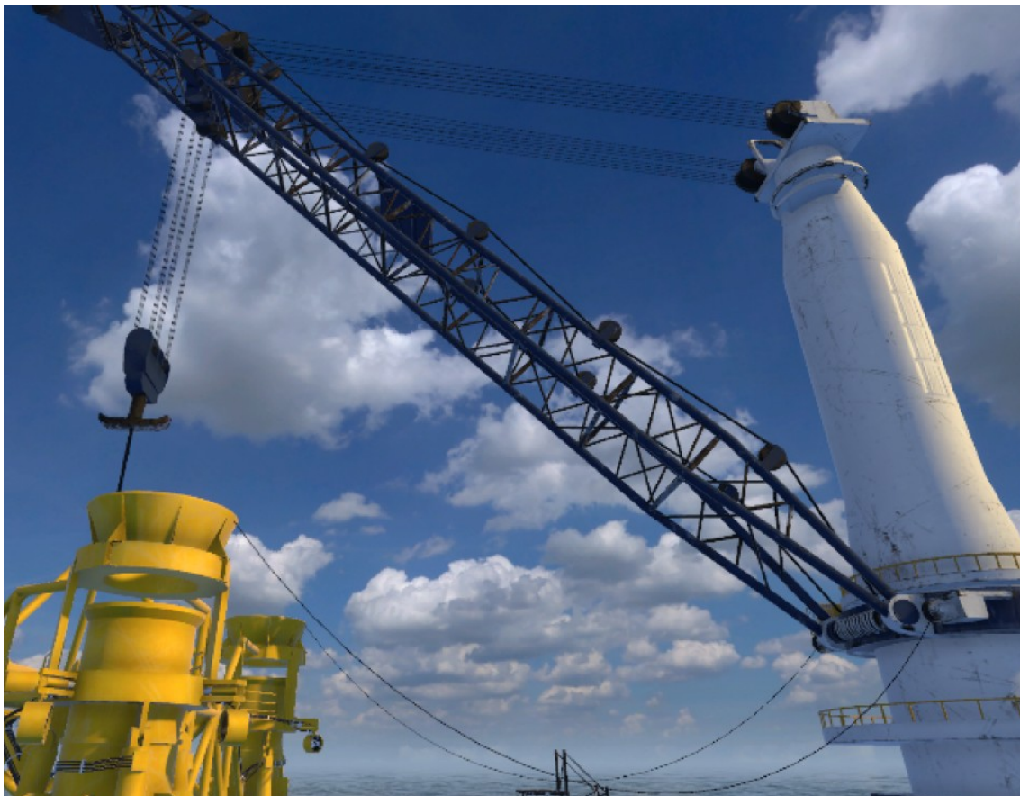
Figure 9: Crane loading the template with the main hoist and tugger lines.
